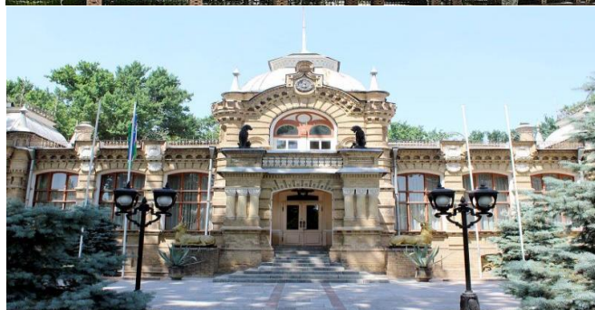
The headquarters of the Prince Romanov is one of the most exclusive architectural constructions of Tashkent built in 1891. Its project was famous architect A.L. Benua and V.S. Belongs to the Geynelsman.
